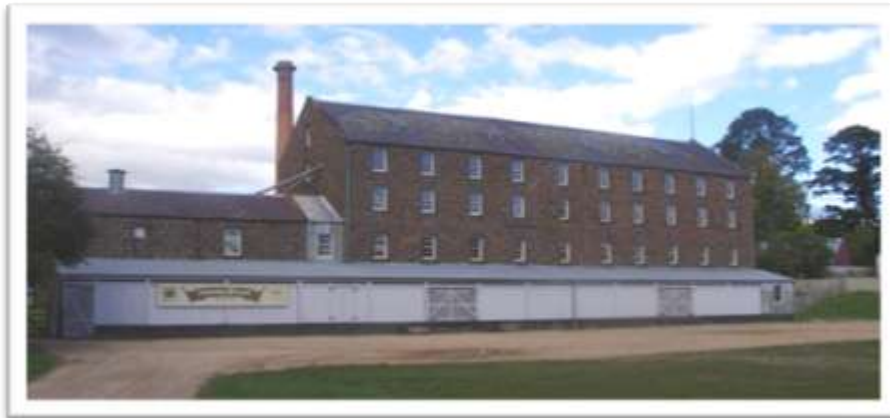
Historic Andersons Mill Smeaton
